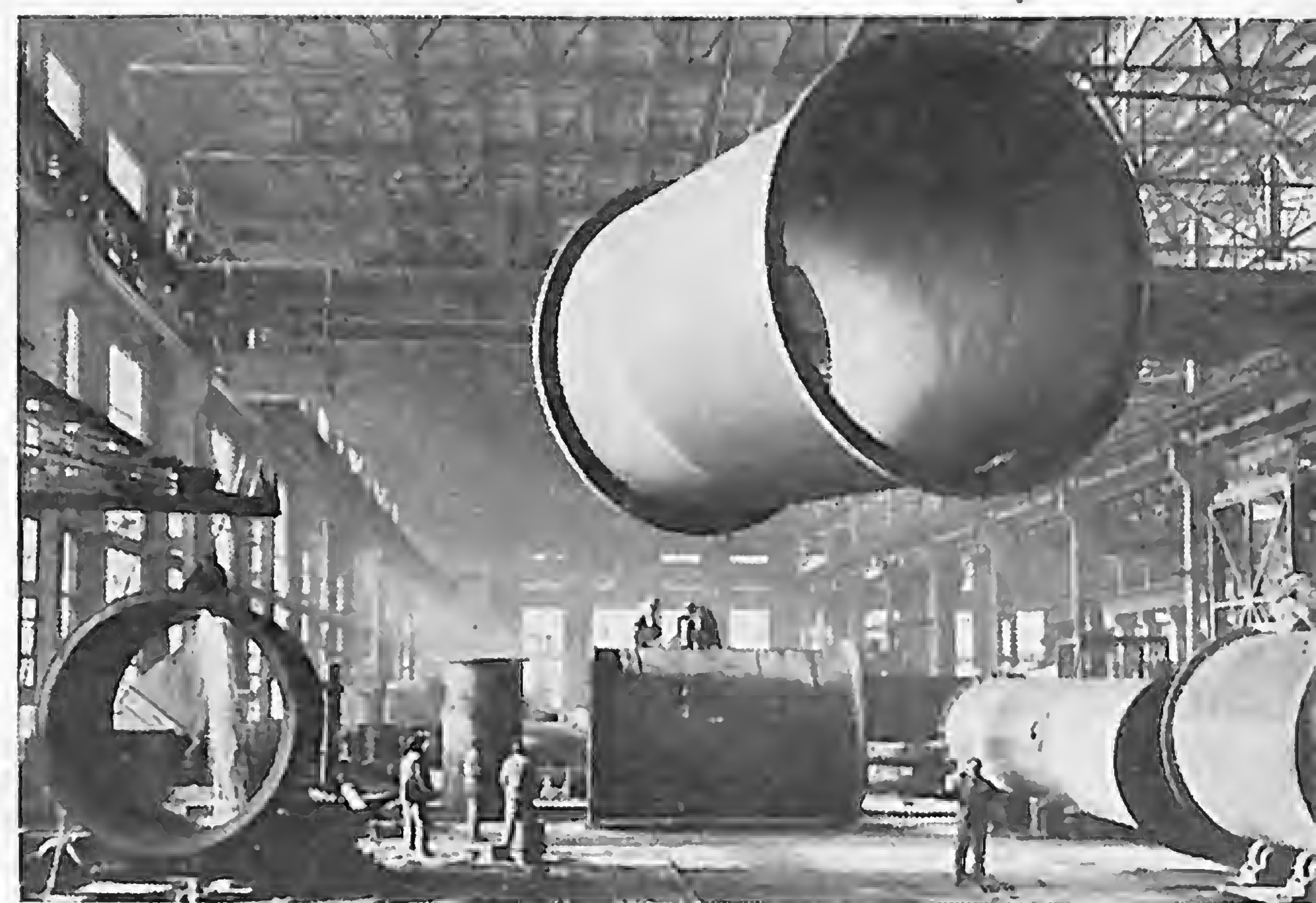
Relying on their own efforts, in seven months the workers and staff of the plant built a riveting and welding workshop with a floor space of 14,000 square meters.
